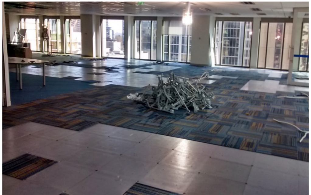
a. Open plan design of an office building after demolition
