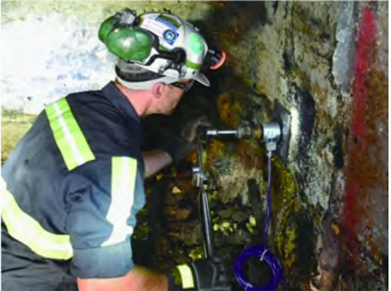
Fig. 3. An installation torque is applied manually to the bolt.
