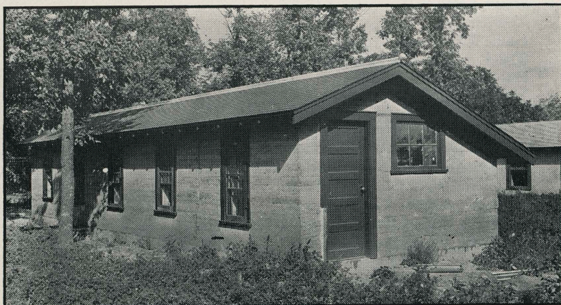
Fig. 1—A 14x40 FOOT RAMMED EARTH STATIONARY BROODER HOUSE These walls are made of very favorable soil containing 75 per cent sand. The building was constructed on the poultry farm at South Dakota State College in 1936. The building is reasonably fireproof. The walls are entirely fireproof.
