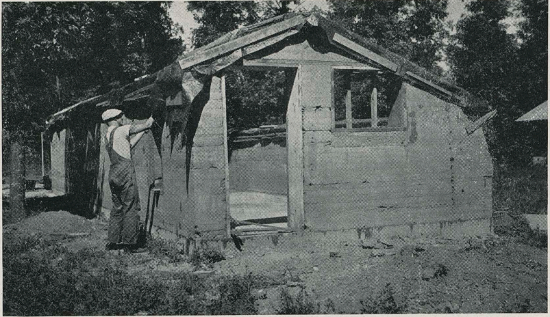
Fig. 15—PROTECTING THE TOP OF RAMMED EARTH WALLS DURING CONSTRUCTION
