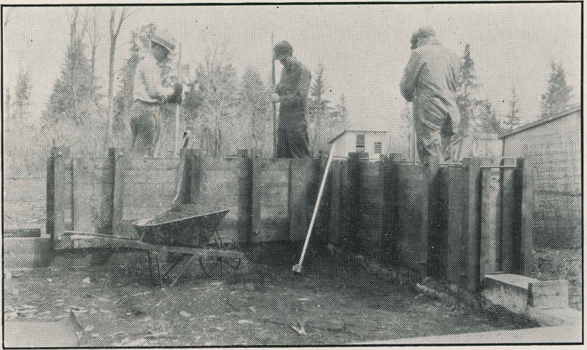
Fig. 13—RAMMING THE FIRST CORNER SECTION OF THE POULTRY HOUSE
