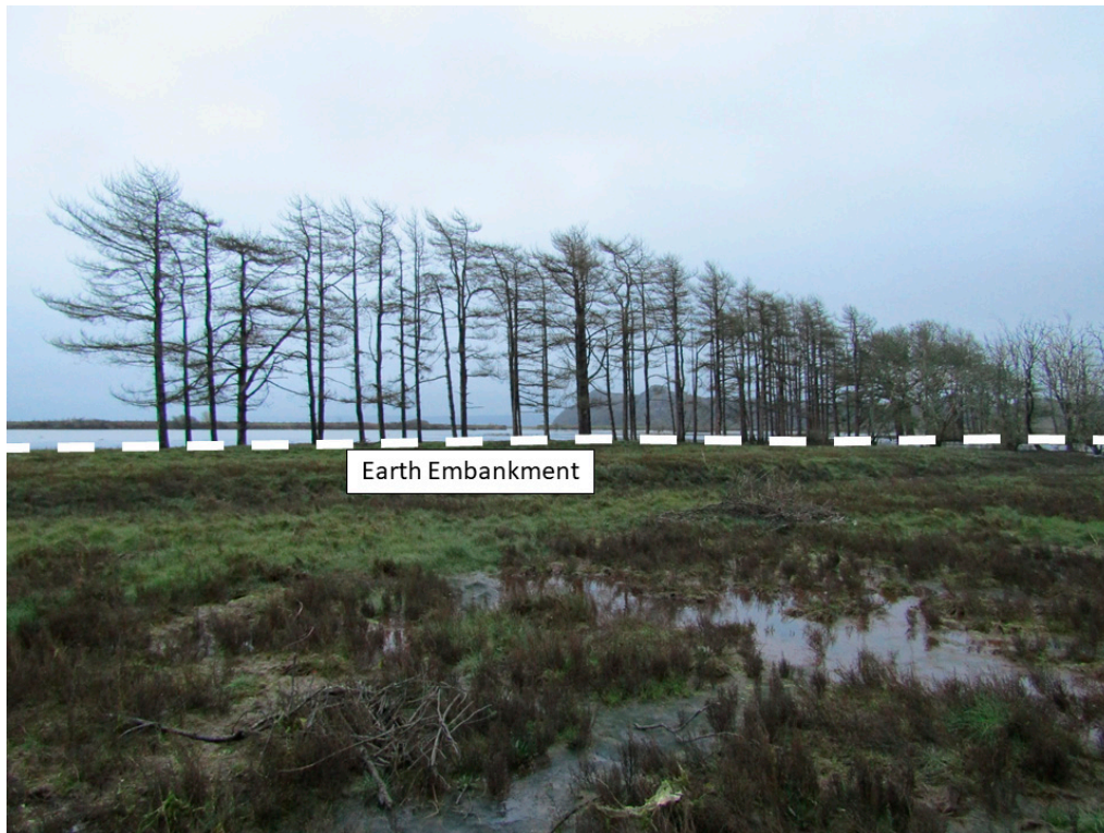
Figure 3. The tree-lined earth embankment which divides Zone 2 from Zone 3, marked by the white dashed line and labelled. The photograph was taken looking south-east towards the breach area across Zone 2 into Zone 3 (photography: H. Burgess).
