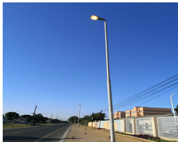
Figure 2: Street lighting switched on in the morning at the National Road 4 (N4) (source: author, May 2020)
