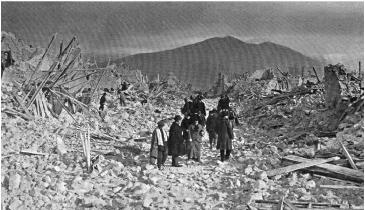
Figure 2. 1915 Avezzano earthquake – damage in Via Napoli [10]
