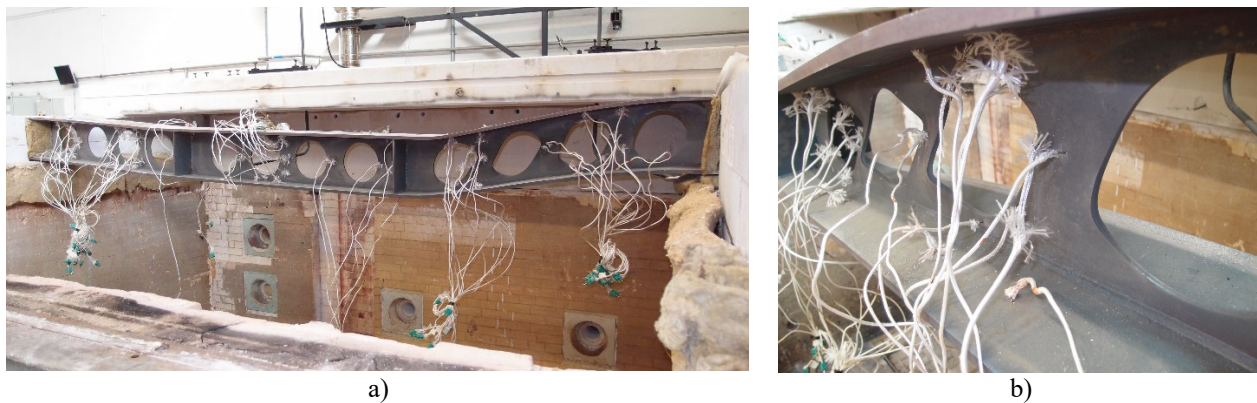
Fig. 4. a) Steel beam after testing; b) Web post buckling failure mechanism
