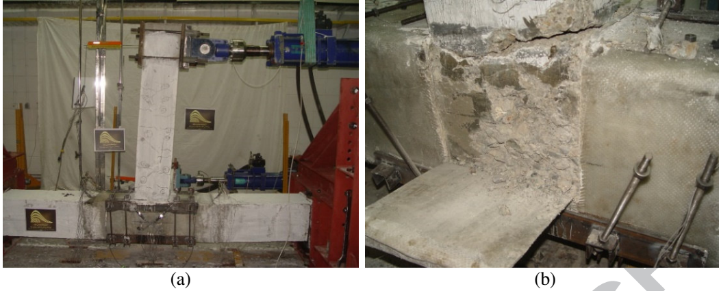
Fig. 10. Distribution of the cracks and damages at the end of the test in specimen TSR: (a) flexural cracks distributed along the length of the vertical beam; (b) crushing of concrete beneath the GFRP composite.
