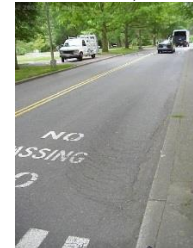
Slippage cracking (Washington Asphalt Pavement Association, 2018)
