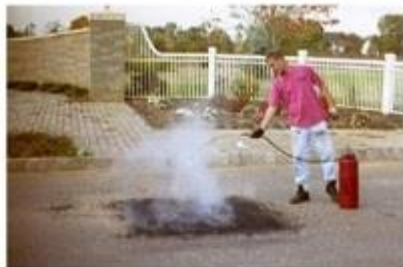
5. Application of rejuvenator to reinstate the properties of old asphalt mixture
