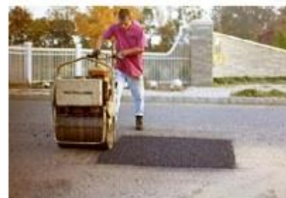
8. Compaction of edges firstly and then inner part
