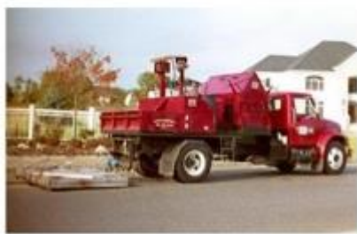
6. Pre-heating of old pavement
