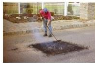
4. Scarification of old pavement
