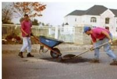
7. Mixing old and asphalt materials
