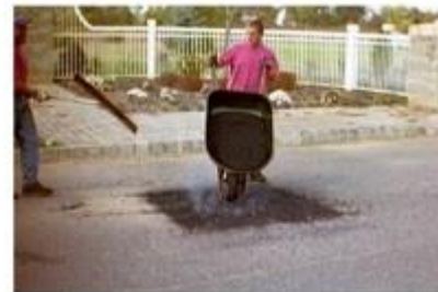
6. Filling with new HMA
