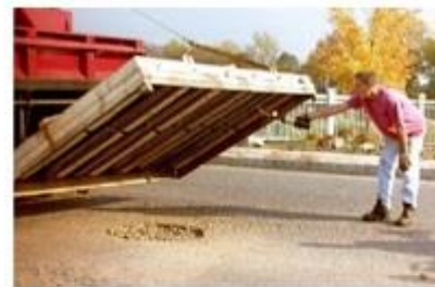
2. Setting-up of infrared heater
