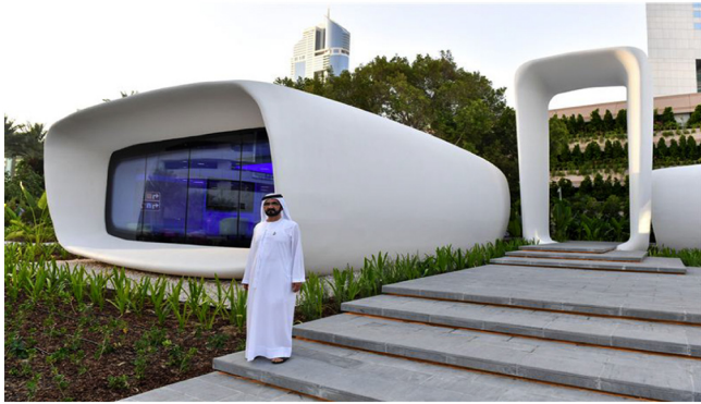
Fig. 3. Office building in Dubai printed by WinSun.
