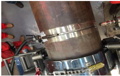
Fig. 14 Narrow Gap weld in SubSea 7 Lab joining of both pipes
