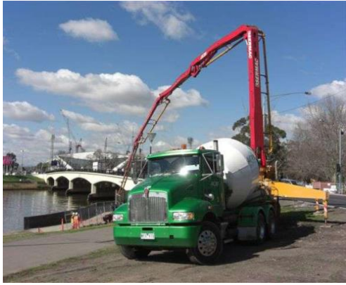
Fig. 2-5 In-situ casting of alkali-activated concrete (ACM, 2009)
