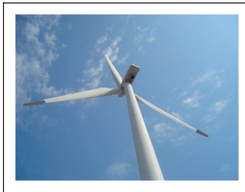
Figure 1. Wind turbine NM750/48 at CRES wind farm in Lavrio (Greece).
