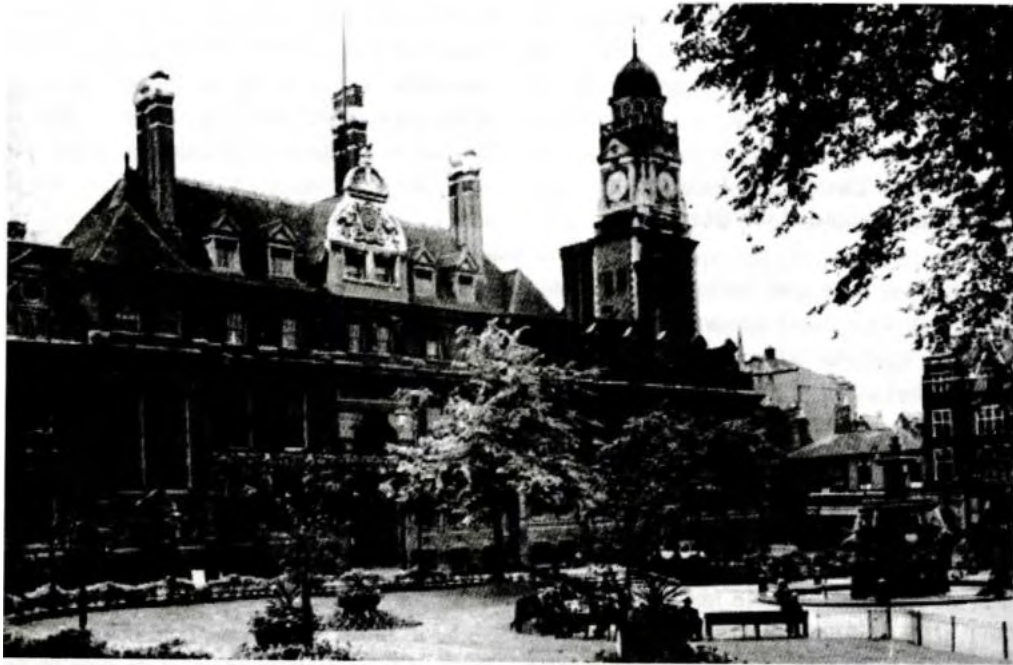
Figures 4. Leicester Town Hall's front elevation as seen from Town Hall Square
