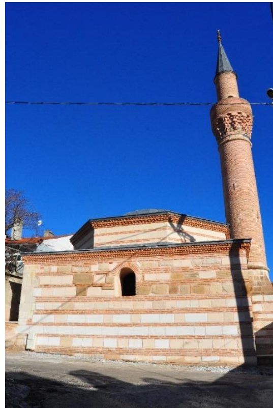
(b) South façade
