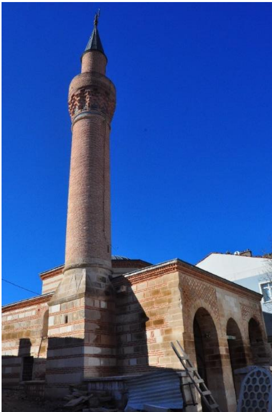
(a) North-East façade
