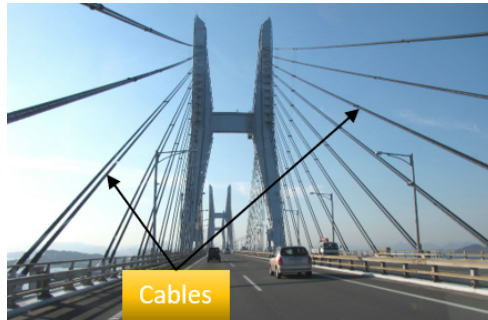
Figure 1.1: Cable-stayed bridge with cables attached at its ends (Picture Information: Signature Bridge, New Delhi retrieved online from [1])
