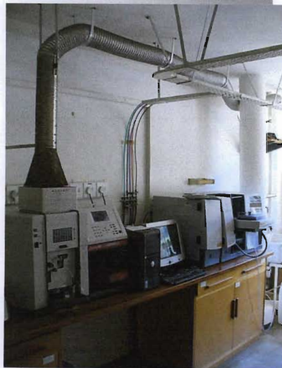
Illustration 5.35: This particular piece of equipment generates exhaust air that is hot. An extraction hood has been installed to exhaust the air to the outside of the building. Similar hoods can be used at individual workspaces. Generally the hood should be wider than the outlet.
