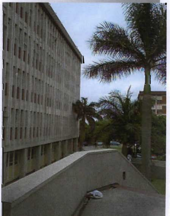
Case Study 3: Block H Laboratories, UKZN Westville Campus
