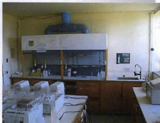
Illustration 5.27: All hazardous processes within a laboratory, especially those generating fumes should be confined to fume cupboards such as the one in the background.
