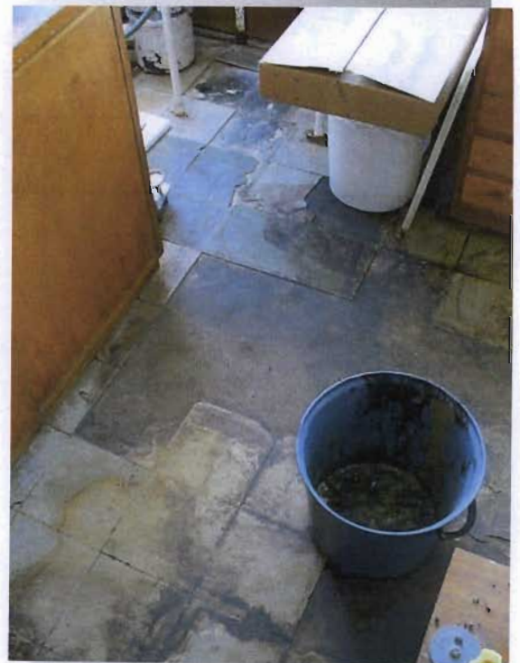
Illustration 5.34: Floor and worktop surfaces need to be particularly durable in a laboratory environment. Generally, vinyl sheet flooring is used with the joints torched, as standard vinyl tiles are inappropriate as spills can penetrate the joints
