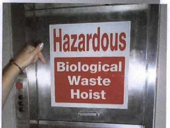
Illustration 5.21: Hoist for transporting biological waste from the upper floors of the laboratory building to the temporary storage facility on the ground floor
