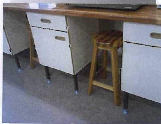
Illustration 5.40: Laboratory fittings are elevated on legs to allow for unrestricted movement of air to minimise the potential build up of dangerous gasses.
