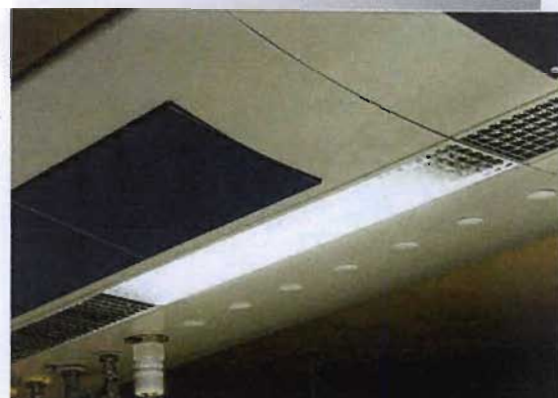
Illustration 7.10: Task lighting is included on the underside of the service carrier to illuminate the directly affected work area. Source: (Waldner Firmengruppe: n.d., 34)
