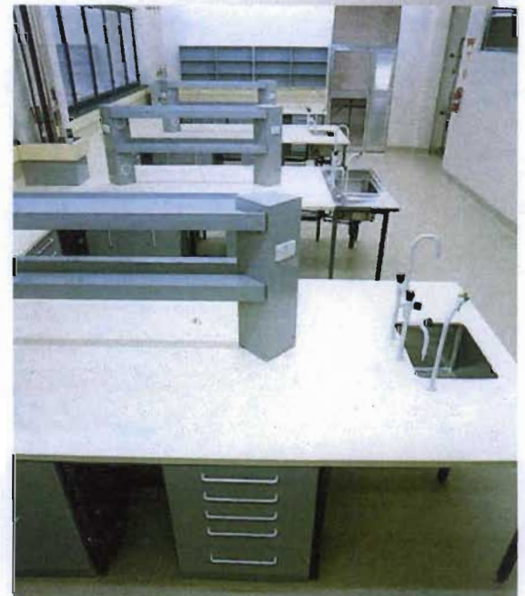
Illustration 7.6: A typical wet laboratory with numerous piped services, sinks and continuous workbenches.
