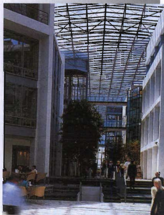
Illustration 2: A view of the internal street in the British Airways HQ offices. Cafeteria seating and vertical circulation open onto the street.
