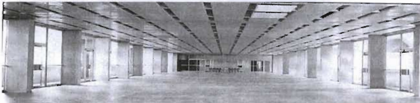
Illustration 4.14: The open plan laboratory space without any equipment or benches. Servicing is from the slots in the ceiling. This allows for maximum flexibility, which the Institute laboratories are praised for. Subsequent plans show that it is subdivided, thus indicating that such a large area is not a necessity.
