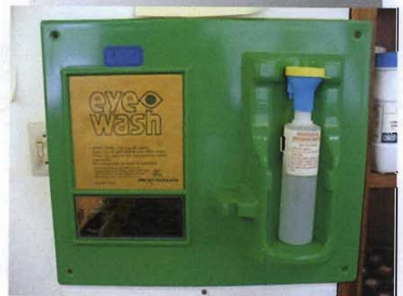
Illustration 7.30: A laboratory eye wash station at the CSIR, Durban campus laboratories. Ideally this should be consolidated with a safety shower.
