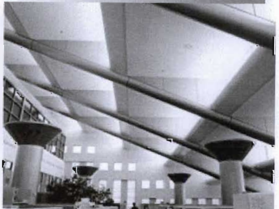
Illustration 7.33: The inclusion of natural daylight is recommended. Not only does it reduce the requirement of artificial lighting, but improves the quality of the space. In the illustrated building, a series of stepped clerestory windows admits natural day-lighting into a large-span space Source: (Wirdzek: 2000, 3)
