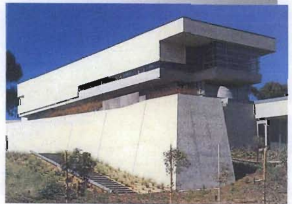
Illustration 4.22: The theory building is situated on a glass ground floor to give the appearance of it 'floating' in response to the way theoreticians operate. Source: (Dietsch: 1996, 90)
