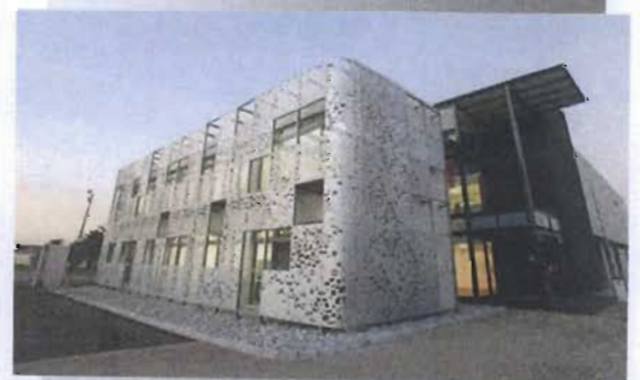
Illustration 1.8: An exterior shot of the BIOVAC building with the prominently screened administration offices in the foreground. During the keynote address at the KwaZulu-Natal Institute of Architects 2007 Awards for Architecture, the Cape Town based architect and winner of a 2007 DaimlerChrysler arts Award, Heinrich Wolff, described it as a building made for the journal photo. Source: (Coetzer: 2007, 89)
