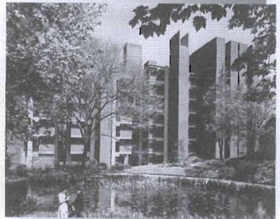
Illustration 3.3: An exterior view of the Richard's Medical Building at the University of Pennsylvania. The prominent vertical brick service shafts are clearly evident.
