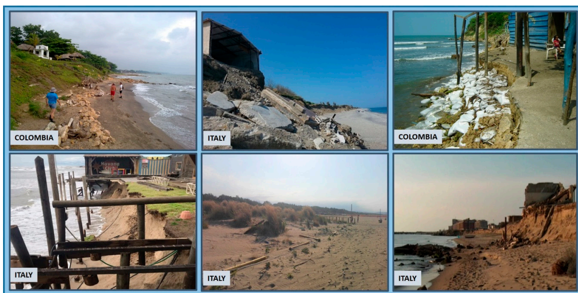
Figure 2. Examples of chronic erosion along low coastal areas in Italy and Colombia. Source: Giorgio Anfuso, Angela Rizzo, Gianluigi Di Paola.
