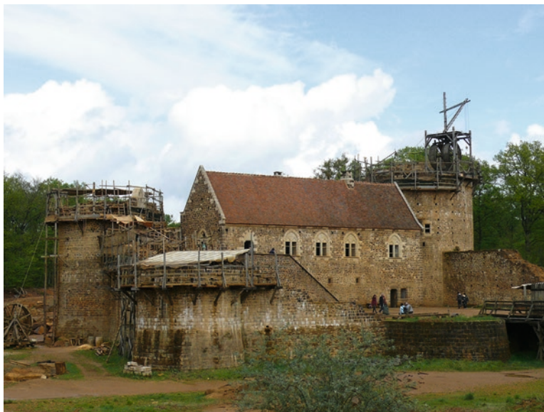
Fig. 4 A thirteenth century castle in the making at Guédelon, central France
