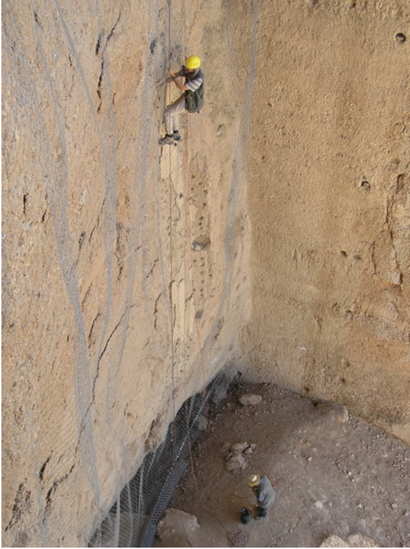
Photo 4 Eastern Buddha, July 2004: Emergency safeguarding of original fragments of clay plaster at the rear face of the Eastern Buddha. (© Bert Praxenthaler)
