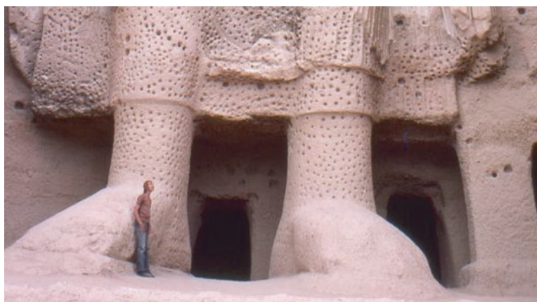
Fig. 5 Situation at the bottom of the 38 m Buddha niche after completion of the India restoration work in 1974 (note the form of the original pillar to the right). (© Wikimedia Commons, Public Domain)
