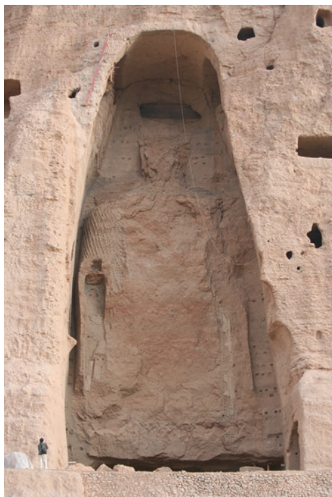
Fig. 8 The rear wall of the Eastern Buddha niche as of 2006 with the remains of carvings and original plaster of the 38 m Buddha figure. (© I.Mayer/RWTHAcde)
