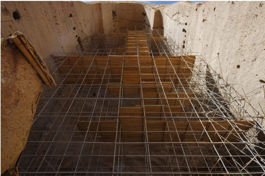
Western Buddha niche with scaffold structure. Situation in October 2015. (© Matthias Beckh)
