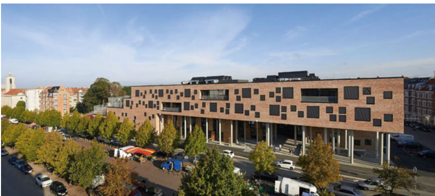
Fig. 2 Impression of the new Frederiksbjerg Skole in Aarhus (DK). Photo and image credits: Henning Larsen, © Hufton+Crow
