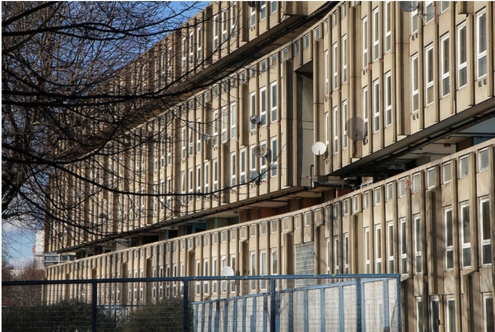
Figure 12 Mikou, A. (2016) Robin Hood Gardens Estate West Block. View from Cotton Street [Photograph]. Unpublished Personal Photograph.
