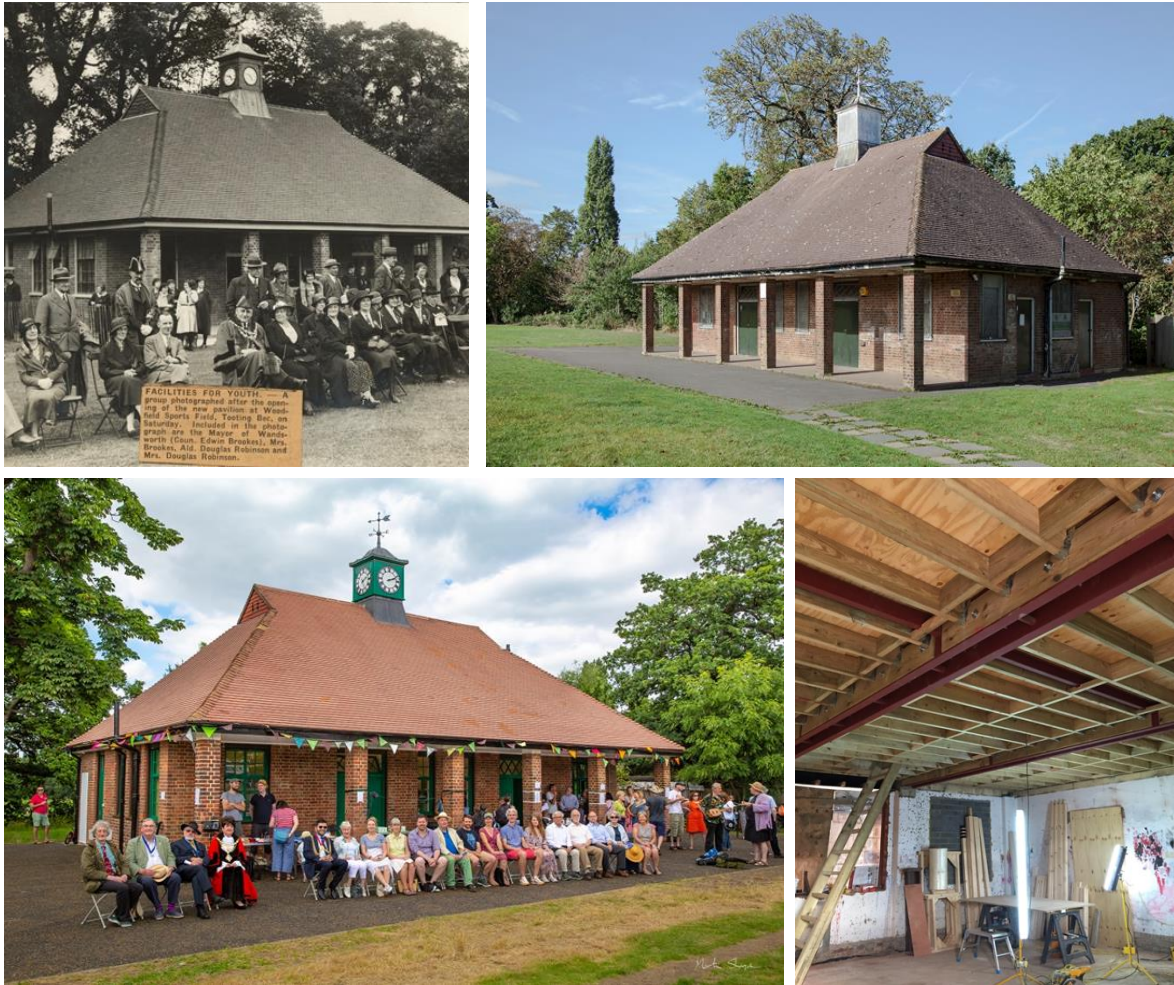
Figure 7 Clockwise from top left: The opening of the Woodfield Pavilion in May 1933, the empty building in May 1918 prior to the start of works, renovation in progress and the opening of the restored Pavilion in June 2019.
