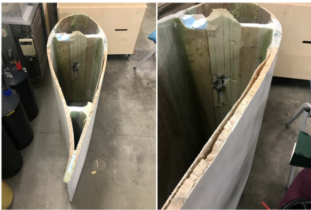
Fig. 3 Sample of defective wind turbine blade showing type 4 delamination detail and area used for the ingress of water during testing. K-band FMCW antenna visible 10 cm to right of structure. Note: delamination situated at internal blade structure and not visible from blade exterior
