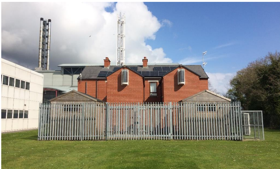
Figure 3-5 Rear of test house on campus. HP and monitoring equipment located in right shed.
