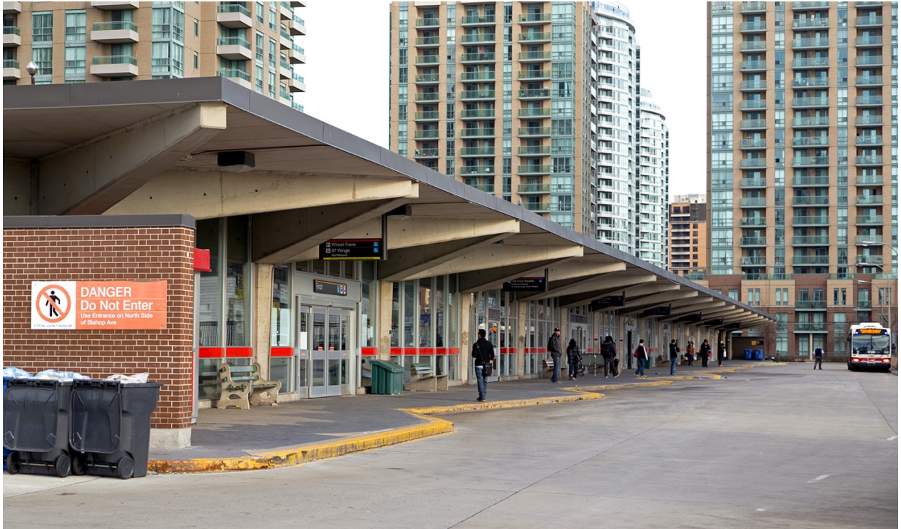
Figure 8: TTC Subway Station Bus Terminal 112
