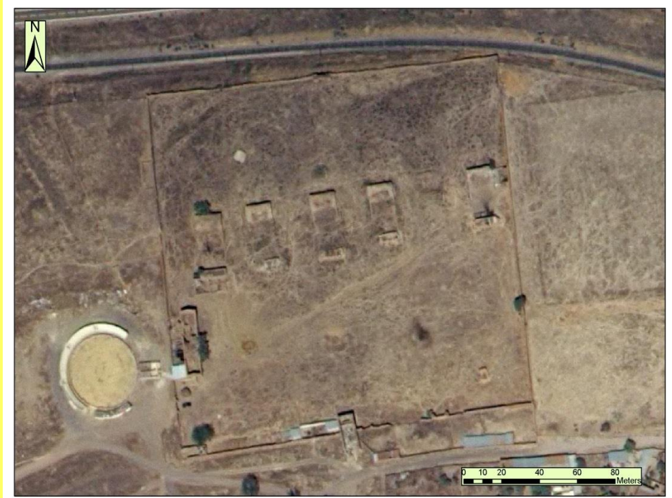
Figure 1. Abandoned metallurgical plant in Almadenejos, Almadén district (R5.5).
