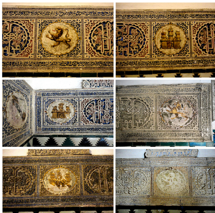
Figure 8 Photographs of the medallions studied in this work showing the different degrees of alteration.
