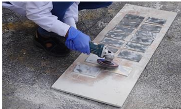
Figure 3.7. Surface Preparation by Grinding of Three-coat System.
