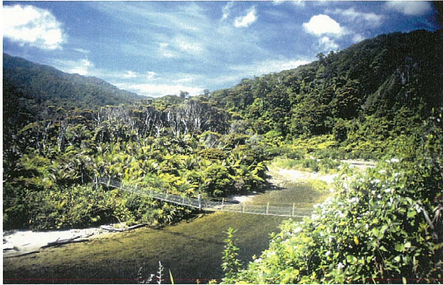
PLATE 8.3: Bridge-crossing on the Heaphy River near the Lewis River confluence NZMS 262-9 (439029) → NE
