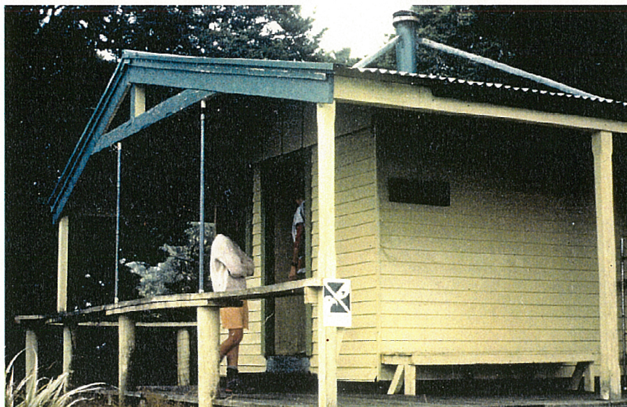
PLATE 7.5: Mount Arthur Hut NZMS 262-9 (486001)→ NE
