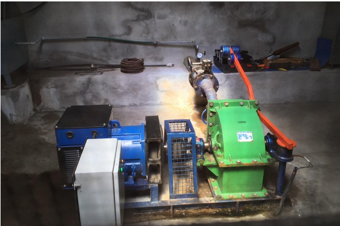
Photo 4: Micro hydro turbine in use in Dovan, rural Nepal.
