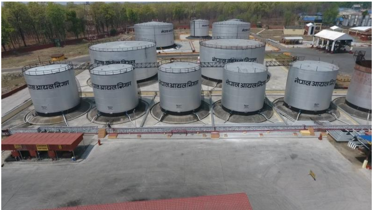
Figure 6.4b: NOC petroleum fuels storage. From NOC (2018e).
