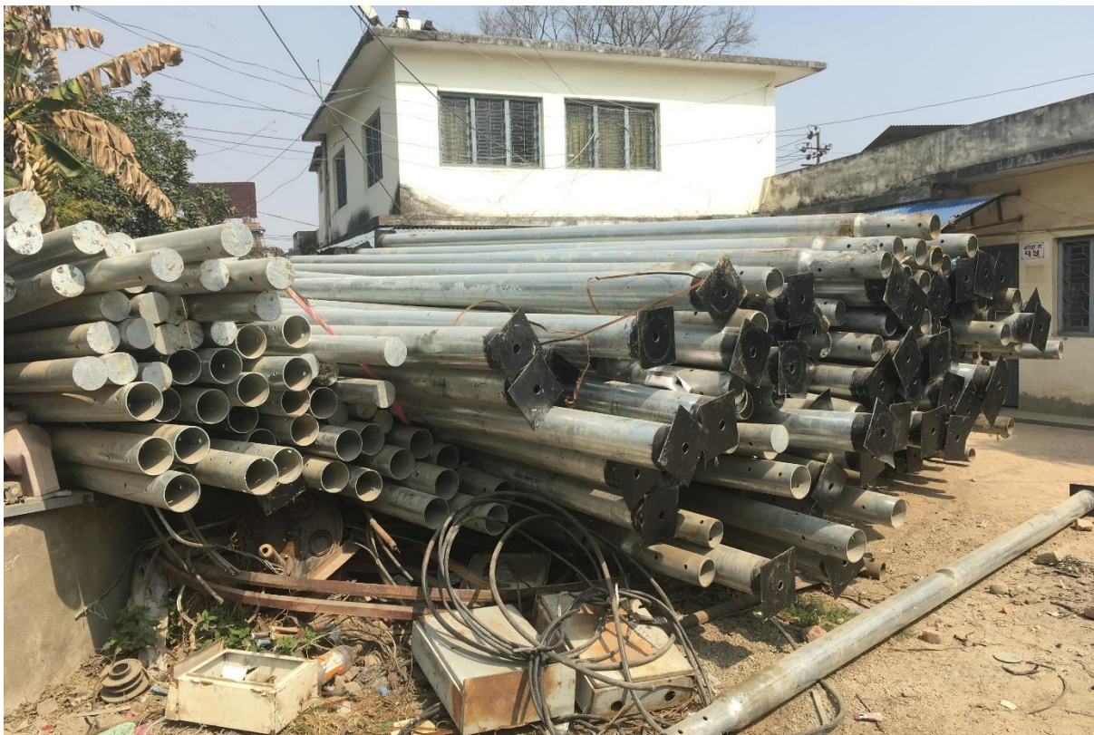
Figure 5.4: Steel poles are being used to replace weaker wooden and concrete poles, which collapsed during the earthquake, damaging lines and cables.
