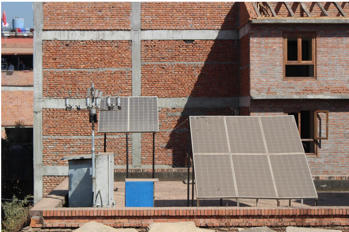
Photo 2: Example of solar panels in Kathmandu. The dust on the panels is an issue as it reduces the panels efficiency.
