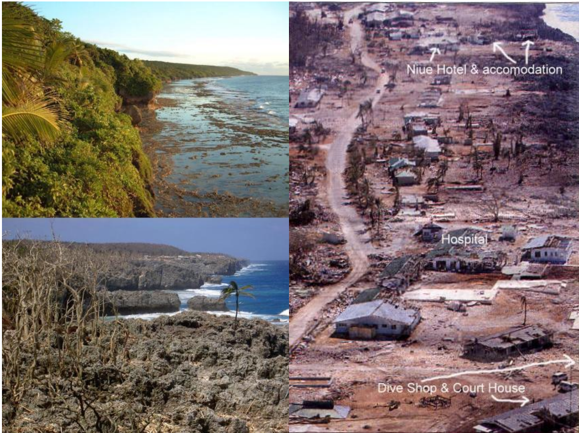
Figure 6.2: Destruction of Cyclone Heta in 2004. Images on the left show before and after the cyclone on Alofi South coastline, the image on the right highlights the buildings destroyed in Alofi South, all of which have been relocated (Source: Niue Yacht Club, 2004).
