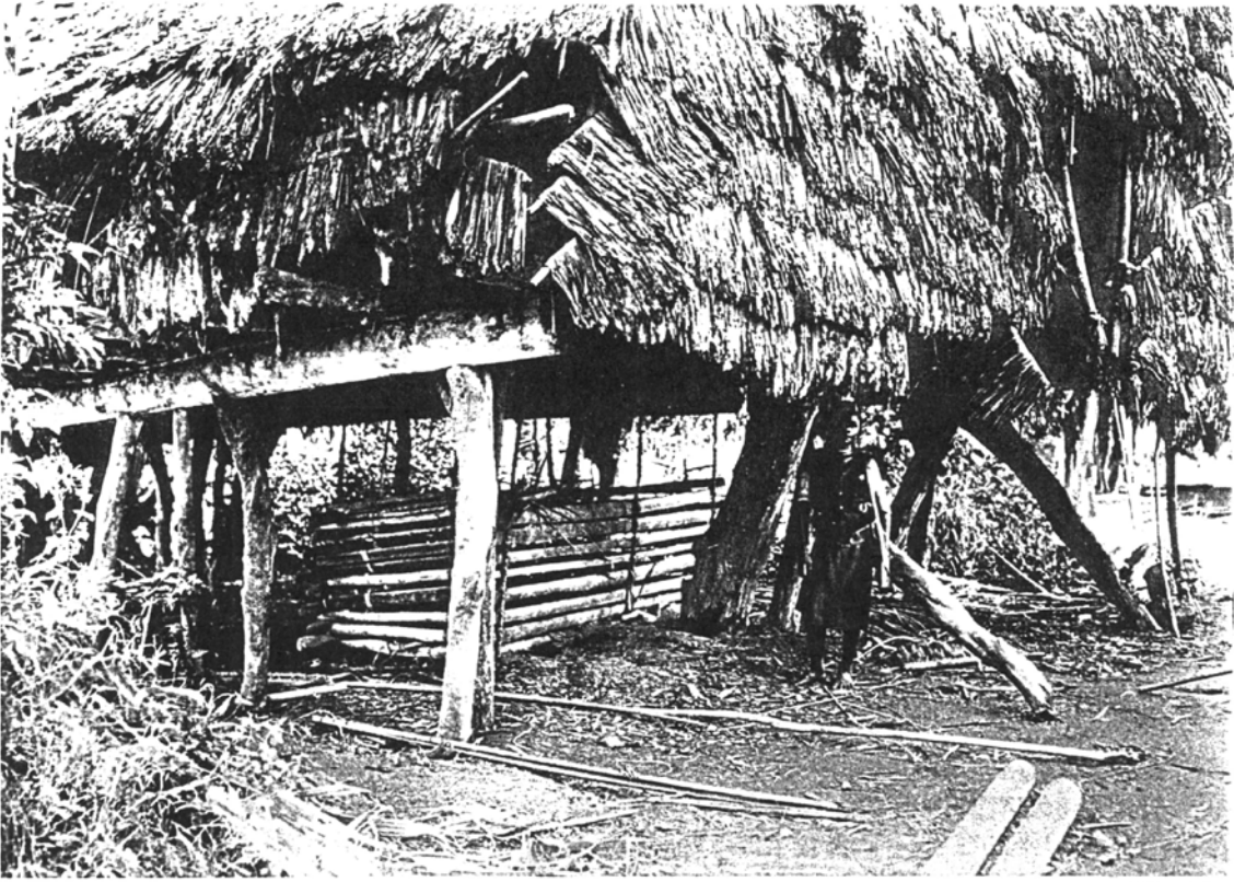
1. A damaged house in Mändānām; a grave beneath it(?) (p. 353)
