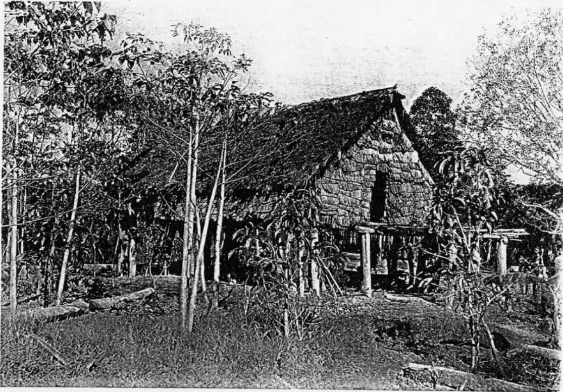
1. Dwelling house, 252 km village (p. 132)
