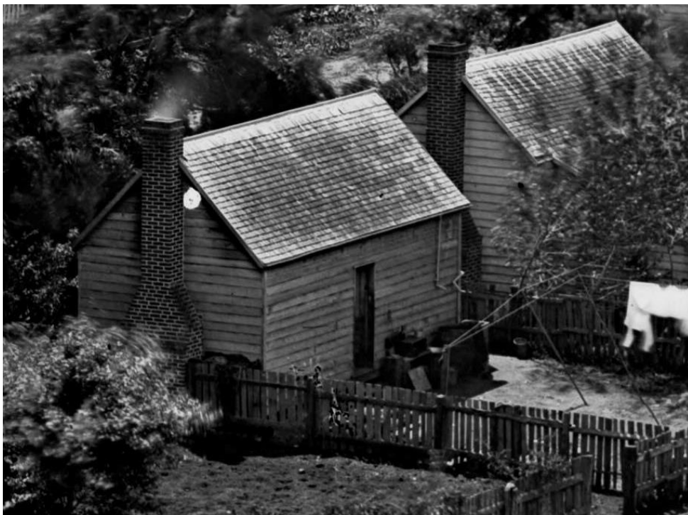
Figure 97. Detail from ca.1870 photograph of Maria Place and St Hill Street corner showing water butt at rear of cottage (right side)
