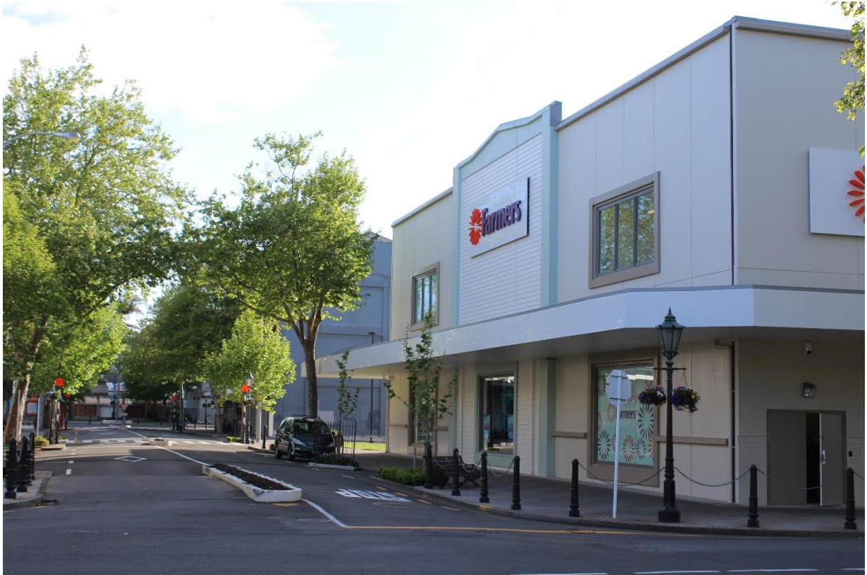
Figure 8. The completed Victoria Retail Centre, October 2016, taken from the Maria Place and St Hill Street corner
