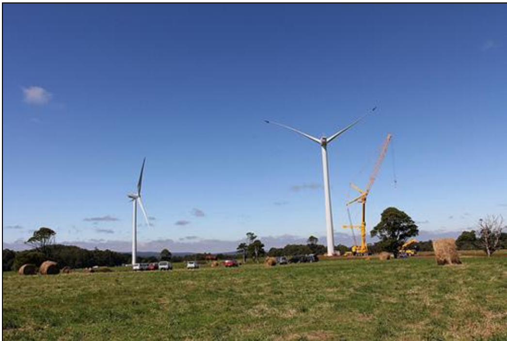
Hepburn Wind Farm during construction, 2011.
