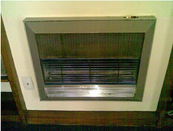
Figure 0.7 Fixed wall heater that wasn't used in H2
