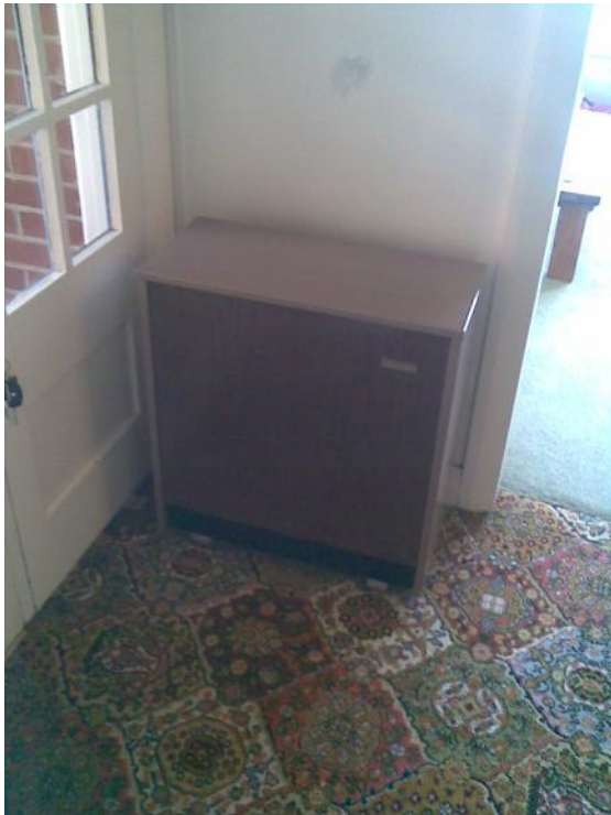
Figure 0.6 The night store heater in the hallway
