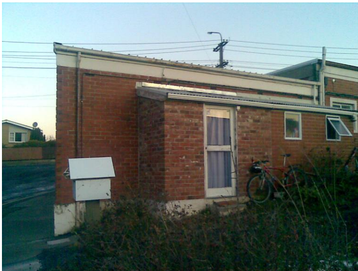
Figure 0.1 Back of the “apartment looking at the bathroom window open
