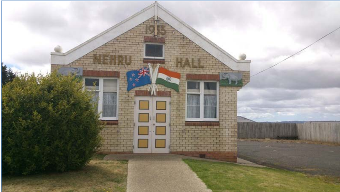
Figure 4. Nehru Hall in Pukekohe, built by the Pukekohe Indian Association in 1953 is no longer used for events as the community has outgrown the venue (Photograph by Alison Booth)
