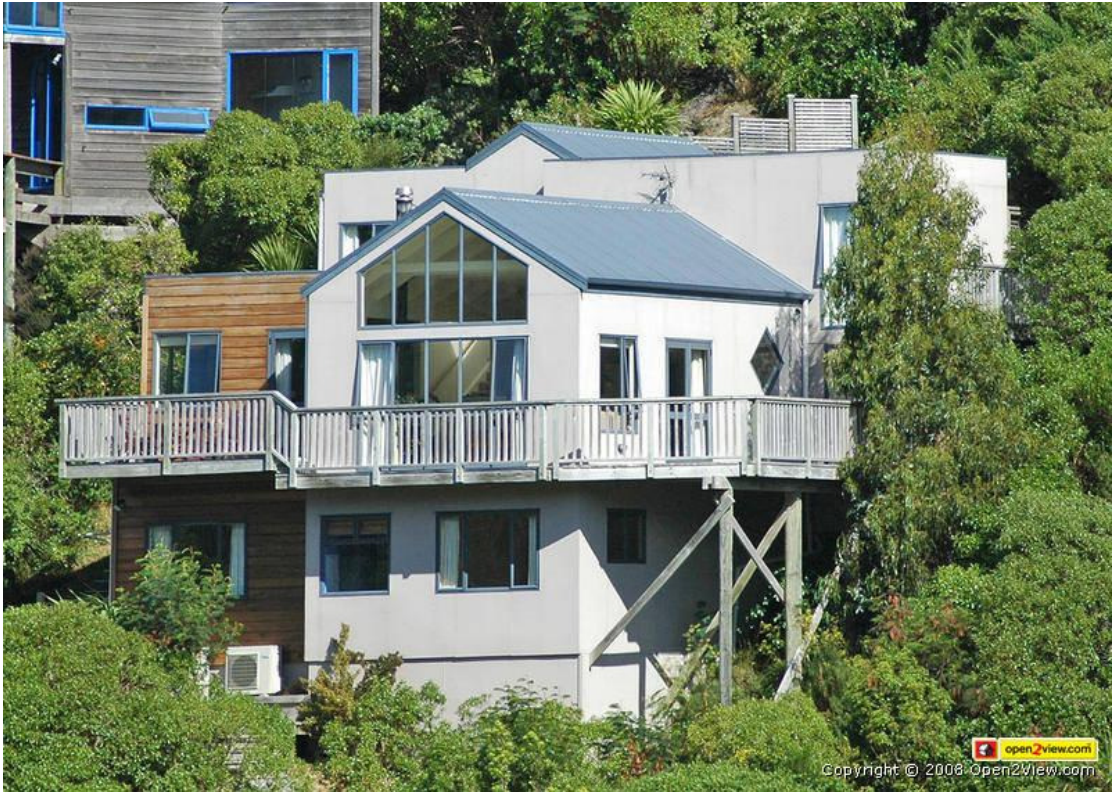
Figure 6.43 1990s Contemporary dwelling, Wadestown, Wellington.
