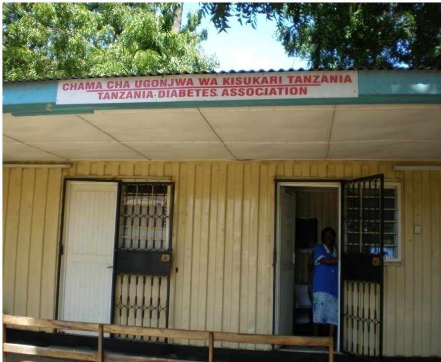
Figure 1.2: Mwnanyamala Diabetes Clinic (refurbished container by Tanzania Diabetes Association), Kinondoni District, Dar es Salaam 2007
