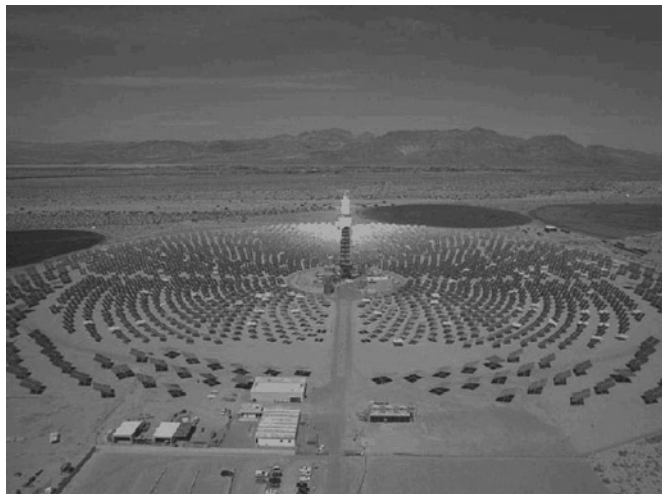
Figure 6: Solar tower with glass mirrors. (National Workshop on "Solar Thermal Power Generation" at IIT Bombay April 28, 2008)
