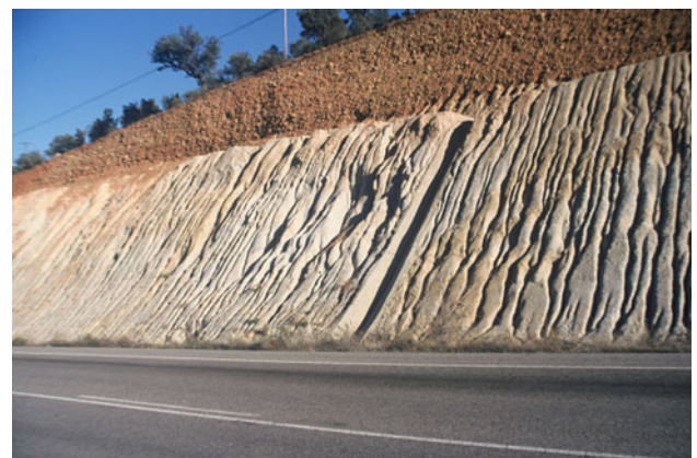
Fig. 5 Clear contact between weathered granodiorite and the Raña cover at the top of the URC profile. The regolith of the granodiorite is very soft and friable and the Raña displays some sedimentary structures in its lower parts
