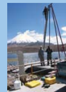
Unloading the platform (left) and setting the tower (right).
