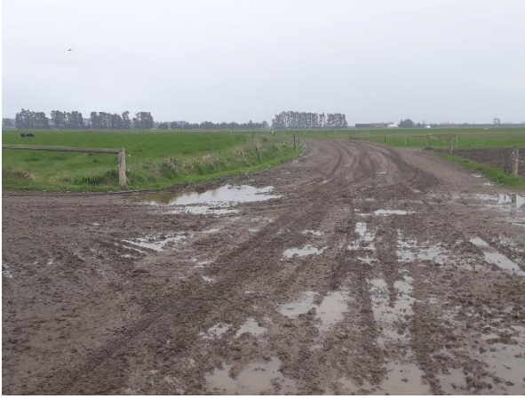
Figure 2.2: Laneway covered in thin layer of mud
