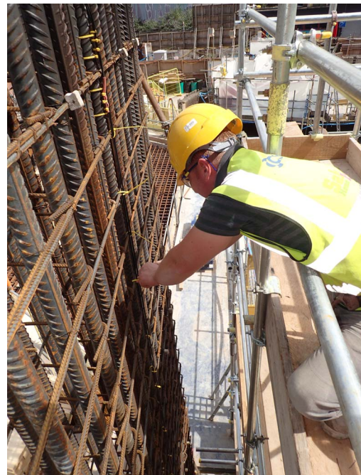
Figure 4 The fibre optic sensing cables being attached to the reinforcement of column C8 before being concreted.
