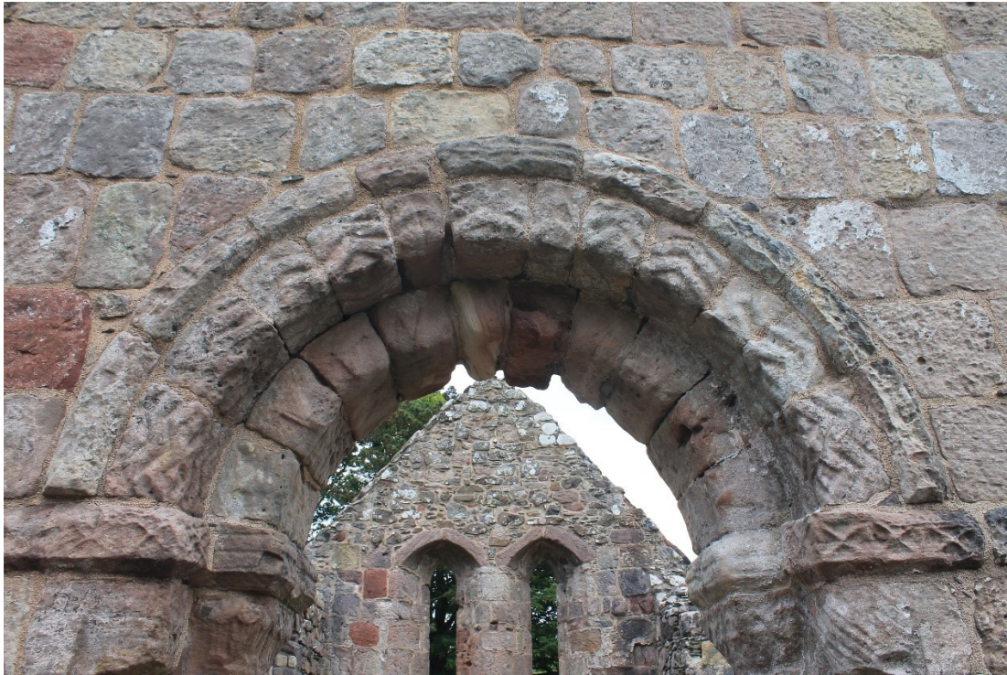
Image 3.1. Kingarth: Romanesque chancel arch with later Northern Gothic rebuilt chancel in background. Note the difference in the shape of the arches and the form of masonry used.
