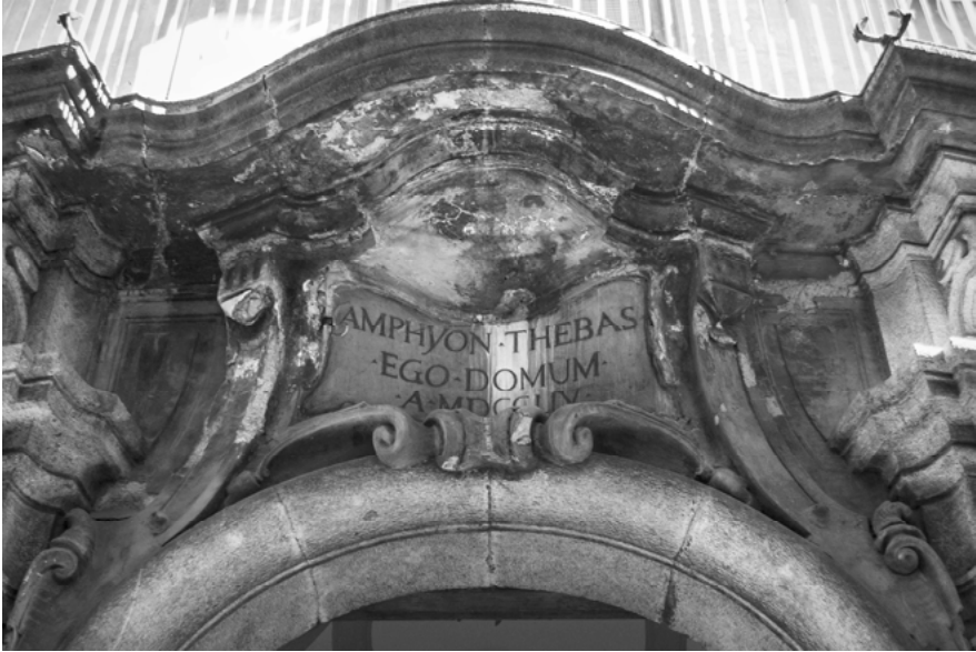
Fig. 2: Portal to the Neapolitan palace of the castrato Caffarelli (Gaetano Majorano, 1703–1783), built in 1754, with a stone pediment that reads “Amphyon Thebas Ego Domum” (“As Amphyon built Thebes, so I built this house”). The building has a pointed arch and upper cornice that function as a balcony for the piano nobile , inside of which is a great staircase with cross vaulting. Photo by Matteo Piscitelli, Naples.
