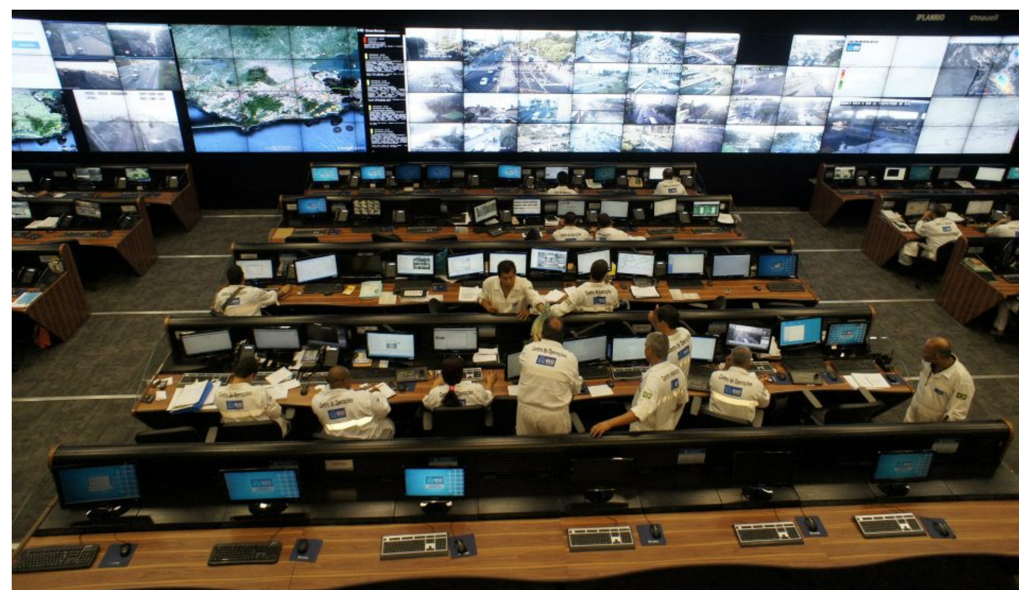
Joint Operations Center
