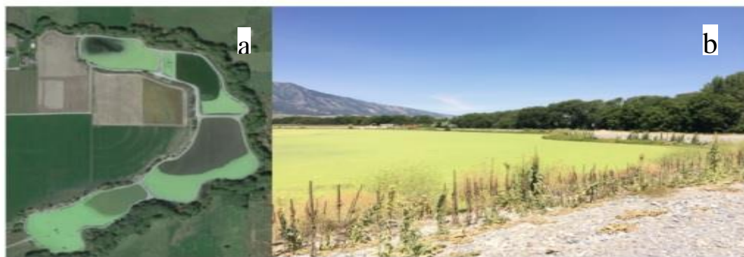
Fig. 3. Wellsville municipal sewage lagoons, Wellsville Utah. (a) Aerial view from Google maps (b) Cell 4 of Wellsville sewage lagoons viewed closely from the north.
