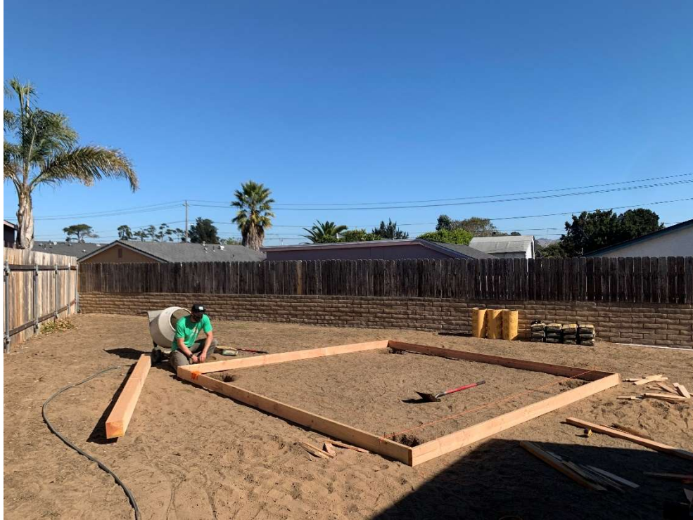
Figure 2: Determining location and verifying measurements are square
