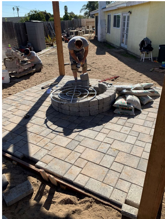
Figure 6: Notching fire ring block to accommodate gas line and valve
