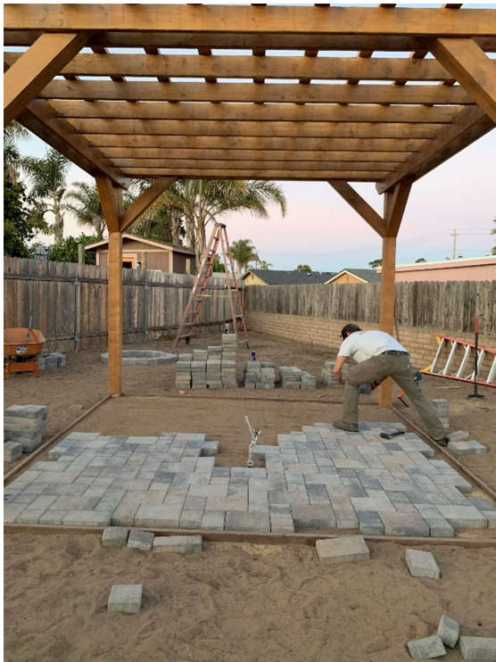
Figure 5: Laying pavers in 1-1-1 pattern
