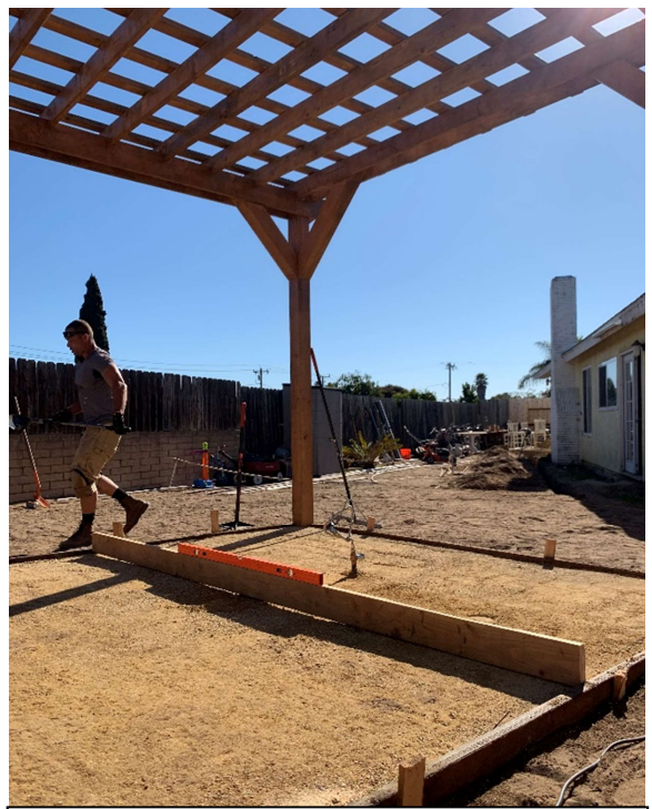
Figure 4: Screeding decomposed granite before and after compacting with hand tamper
