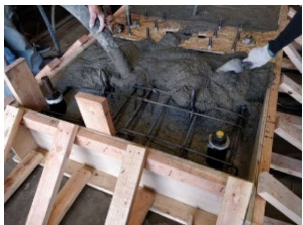
Figure 4-6: Shear Wall Footing Reinforcement (Left) Footing rebar cage and (right) concrete pour.
