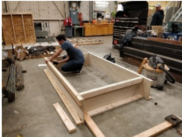
Figure 4-5: Shear Wall Footing Formwork Construction
