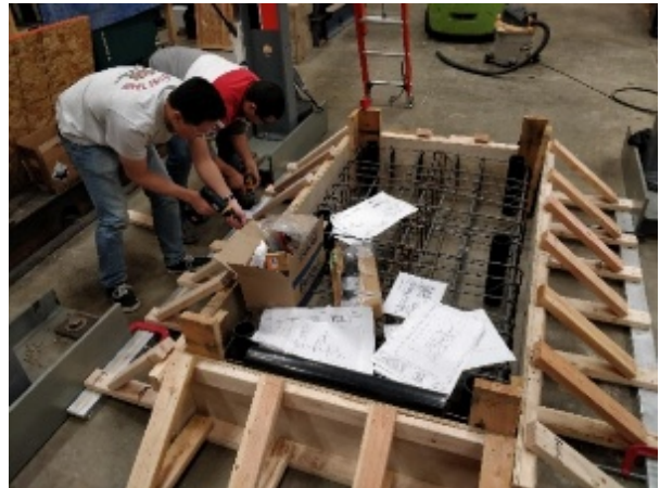
Figure 4-5: Shear Wall Footing Formwork Construction
