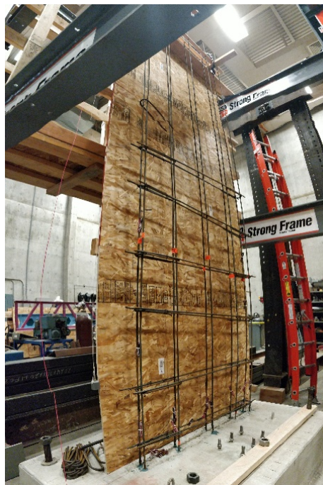
Figure 4-7: Shear Wall Formwork & Rebar Cage Construction
