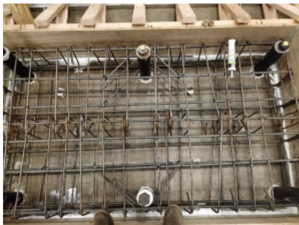
Figure 4-6: Shear Wall Footing Reinforcement (Left) Footing rebar cage and (right) concrete pour.
