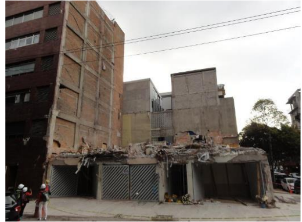
B) Flat slab collapse
