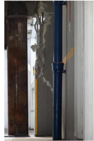
C) Buckling damage
