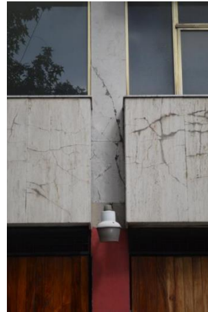
B) Shear damage
